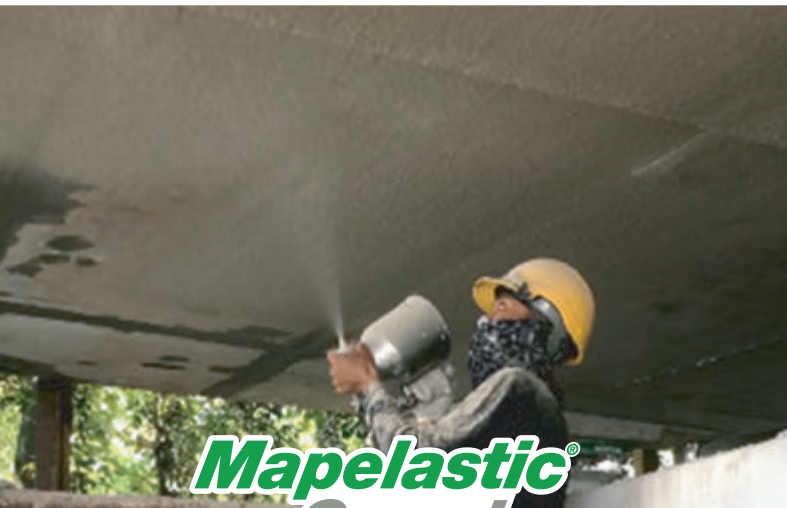
Seri Tanjung Pinang Bridge, Penang
