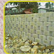
Modular Block Wall Reinforced Concrete Structure
