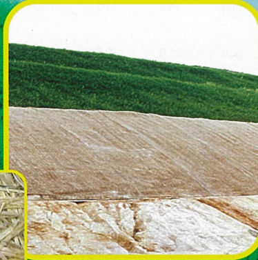
Biodegradable Erosion Control Blanket
