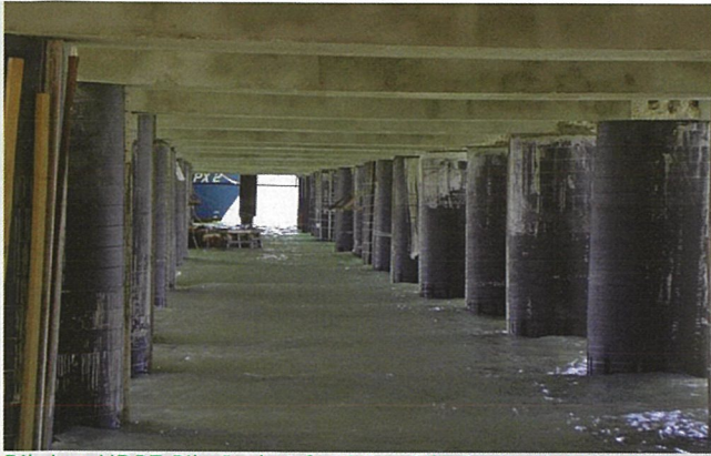
Rib Loc HDPE Pile Jacket for Jetty Pile Protection Work at Pangkalan Polis Marina Langkawi
