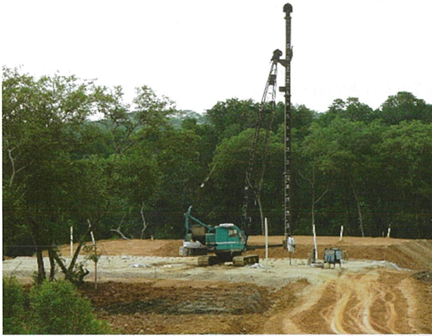
Figure 2: Trial soil improvement before the commencement of filling works
