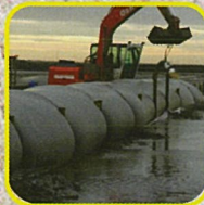
Mega Sandtube Beach Erosion Containment Bund
