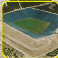
HDPE Geomembrane Area Sealing Application
