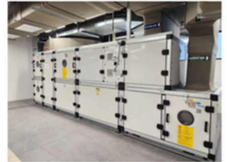
VRV AHU – WITH FULL COMPONENTS: HEATWHEEL, EC PLUG FAN, CONTROL ETC
