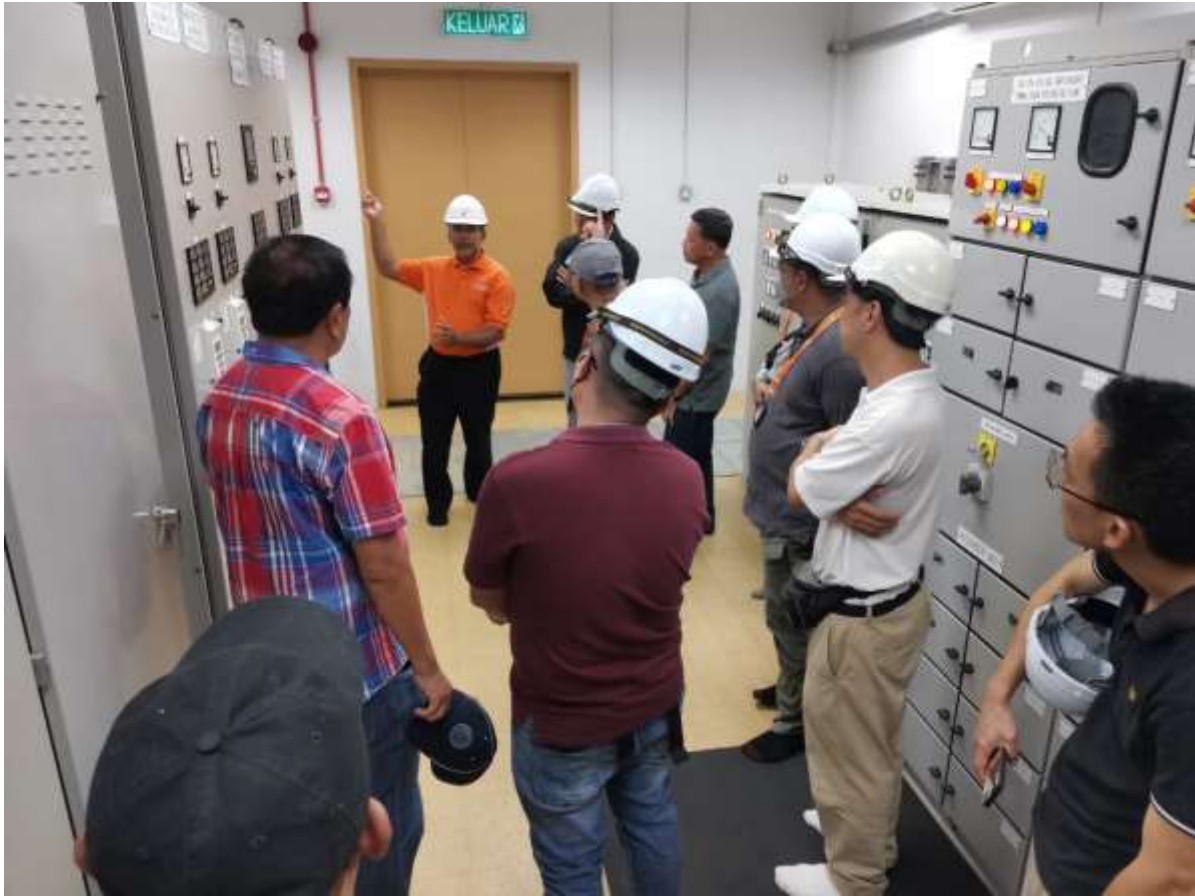
Solar Farm chargeman is giving an explanation for power distribution system
