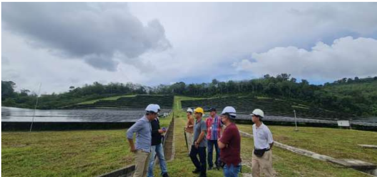
Outdoor solar farm
