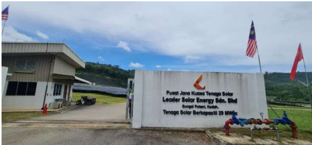
Solar farm main entrance
