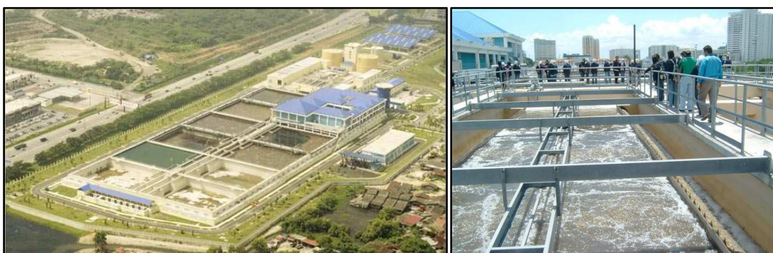
Figure 3.3 : Jelutong Sewage Treatment Plant (1,200,000 PE)
